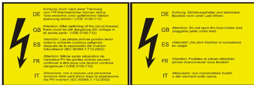
Here is a typical operating equipment label in the enwitec generator junction box
